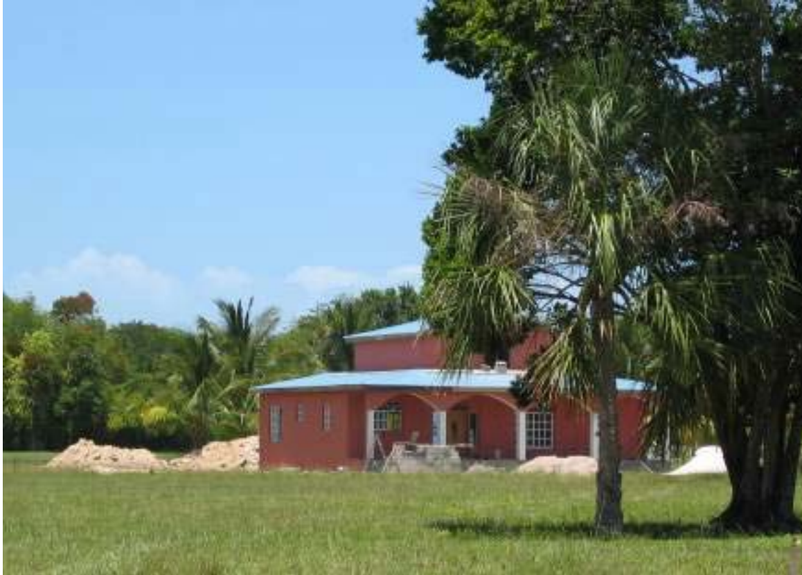
A home under construction at Consejo Shores near Corozal Town
